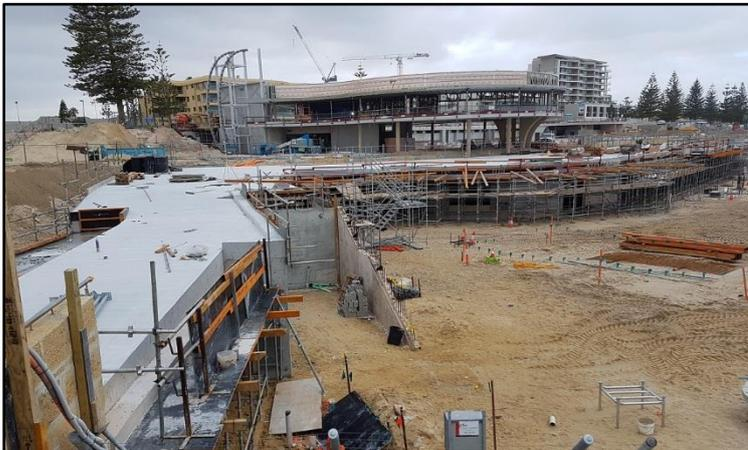
lift for the two story pool restaurant and café complex. Form work for the stairs from the lower promenade level to the beach level is obvious. The shop and kiosk curves around to the equipment store that runs south, parallel to the water line. The pile of structural steel to the right is at the approximate position of the first aid room, Beach Services administration and the new tower.
